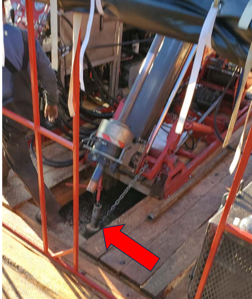
Drill Anchor Set, Ready to Core – DEM23-01
